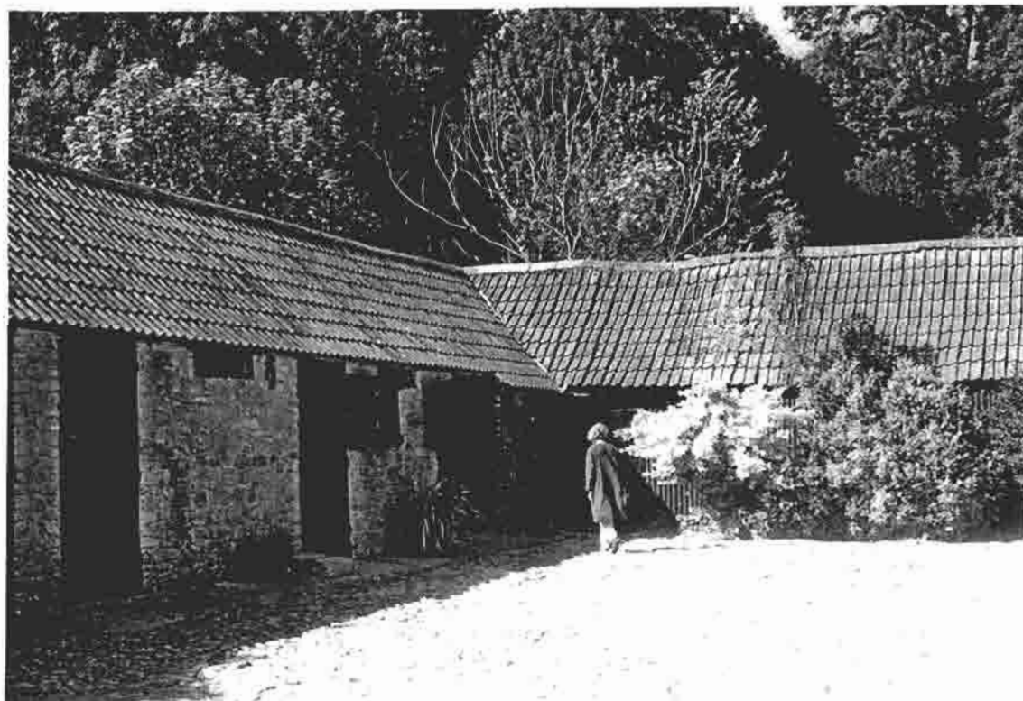
Part of the 19 th century cobbled yard and red pan-tiled ancillary sheds at Uphay, Axminster.
