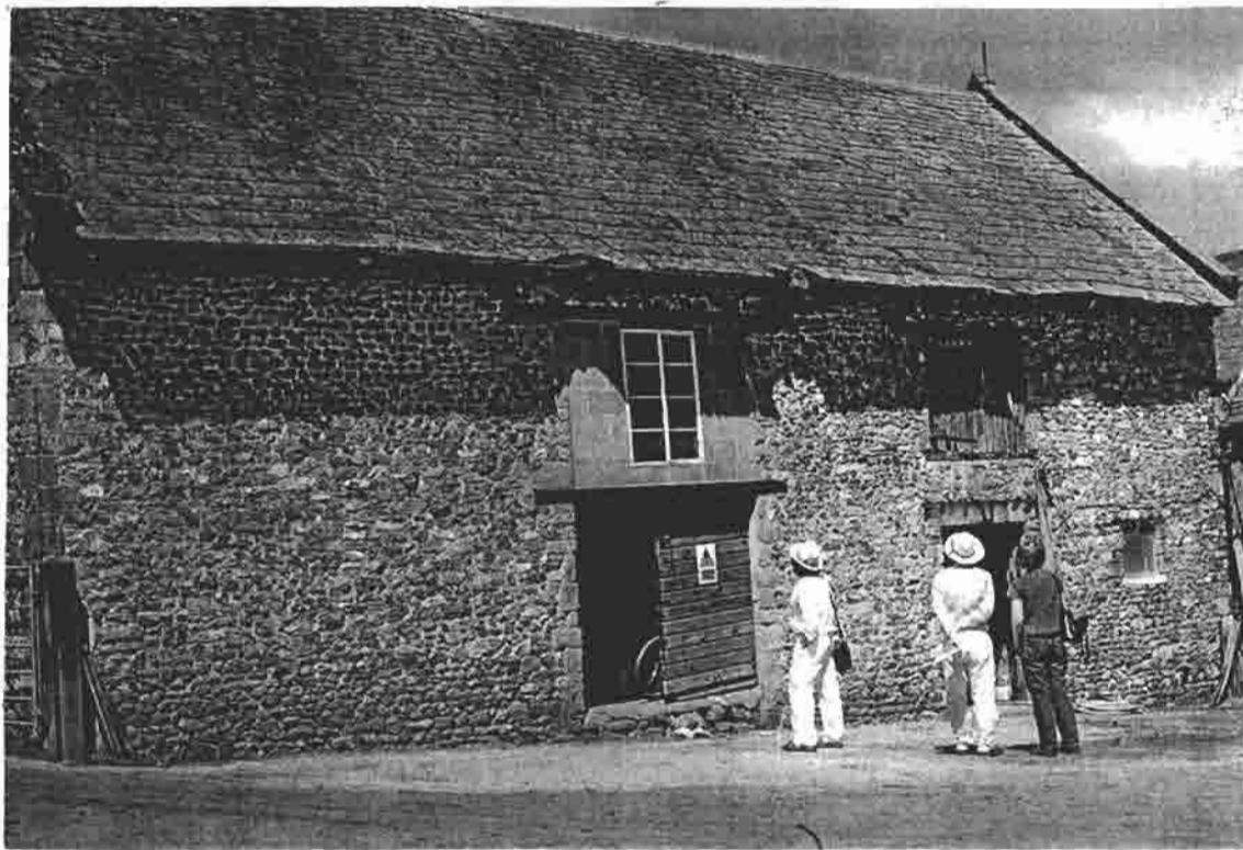
Detached rubble-stone barn with rag-slate roof at Court Place, Yarcombe.
